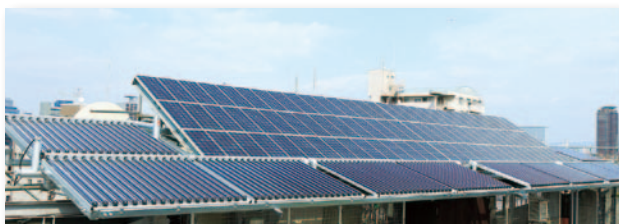
Tube-type, high-performance solar thermal energy collection panel
